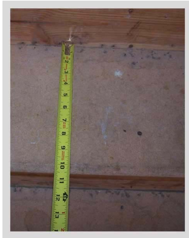
Figure 9: Measuring the stair treads (close-up)
