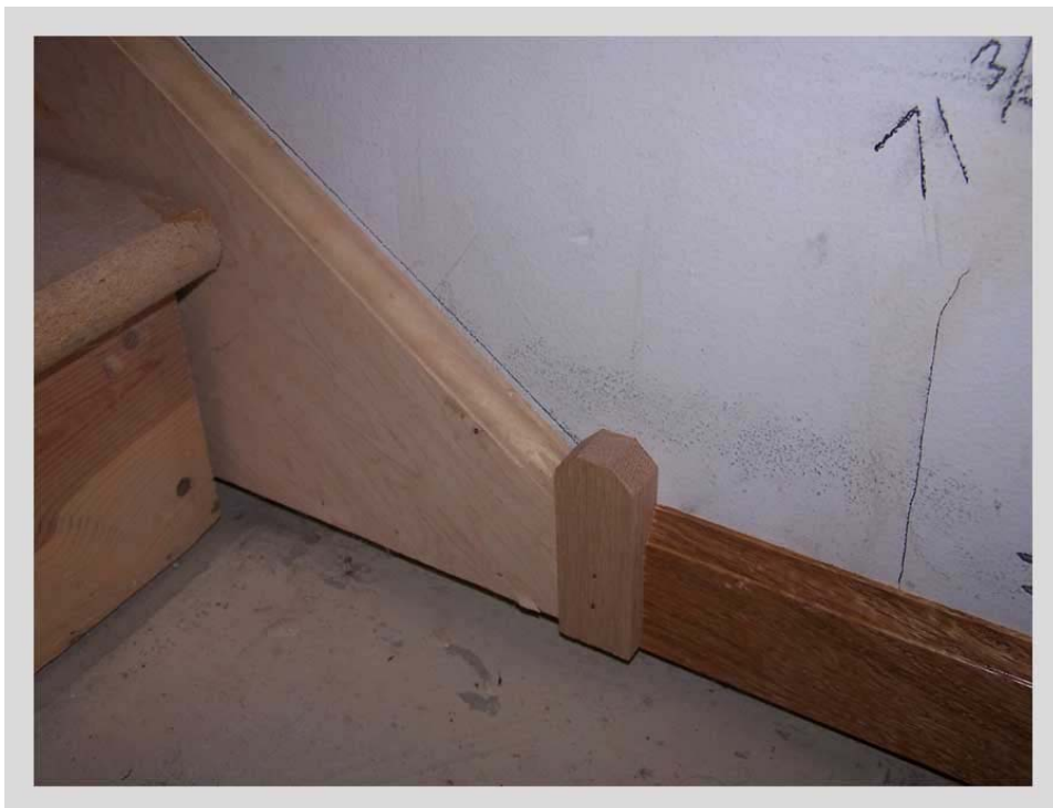
Figure 17: Skirt board fitted (bottom)
