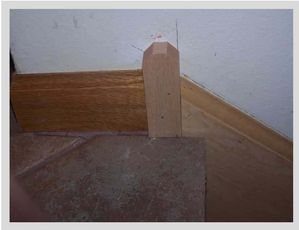
Figure 18: Skirt board fitted (top)
