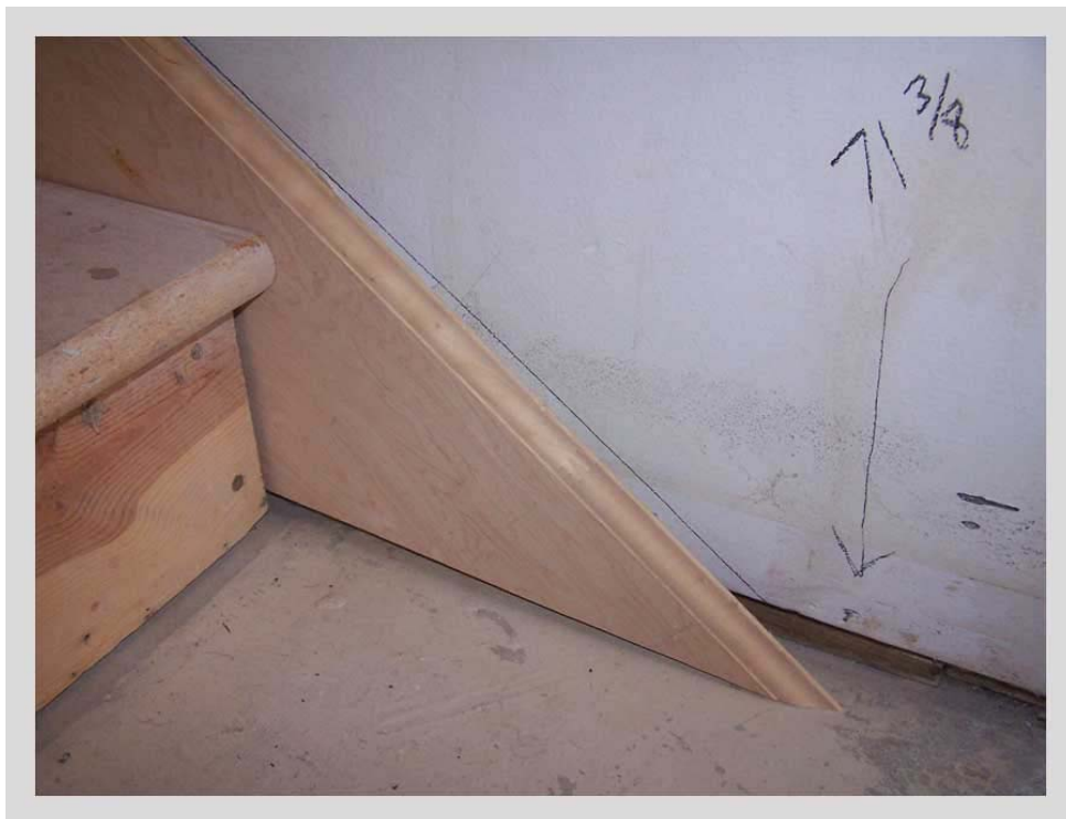
Figure 15: Trial fitting skirt
