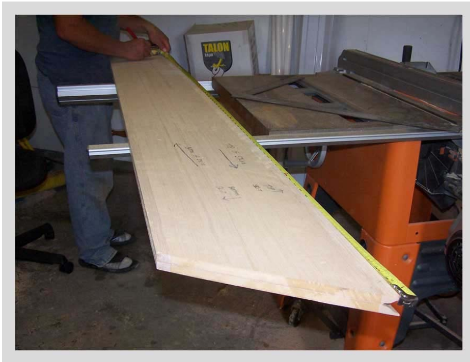
Figure 12: Measuring the skirt board
