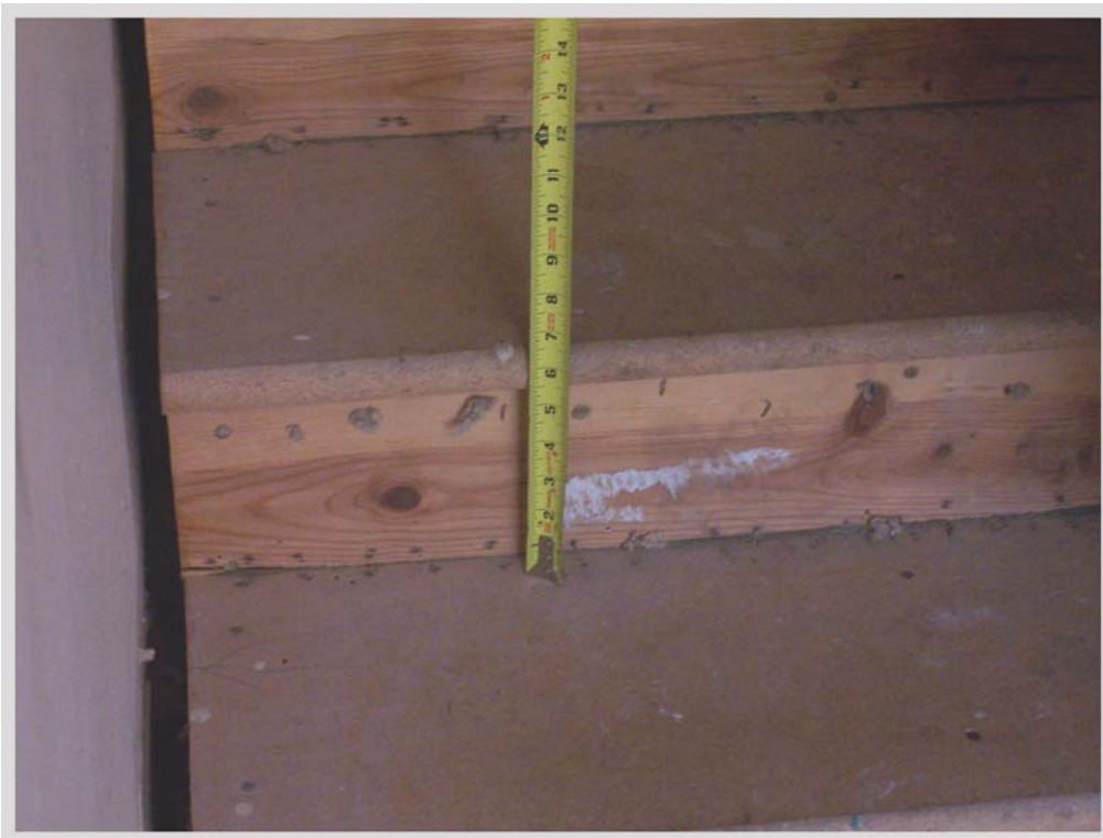
Figure 8: Measuring the risers
