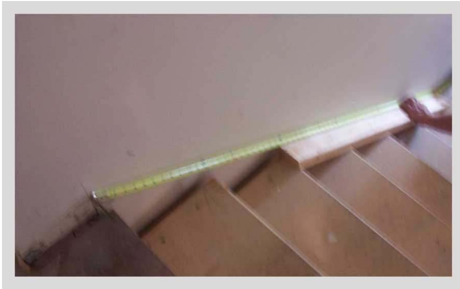
Figure 6: Measuring the length of the skirt
