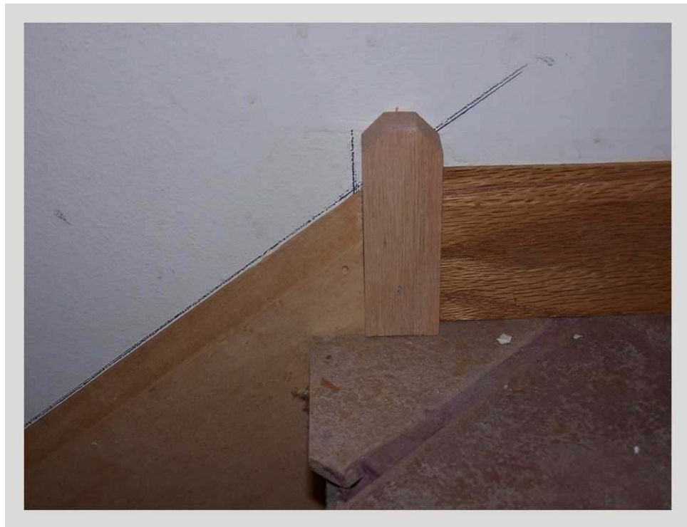
Figure 19: Skirt board fitted (top)
